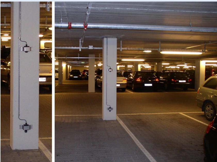
Installation with CO detector and HC detector type GP-SA.
